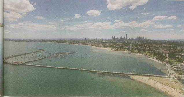
St Kilda Pier A Melbourne landmark since the 1850s, the kiosk was rebuilt to 1903 plans after being destroyed by fire in 2003.
